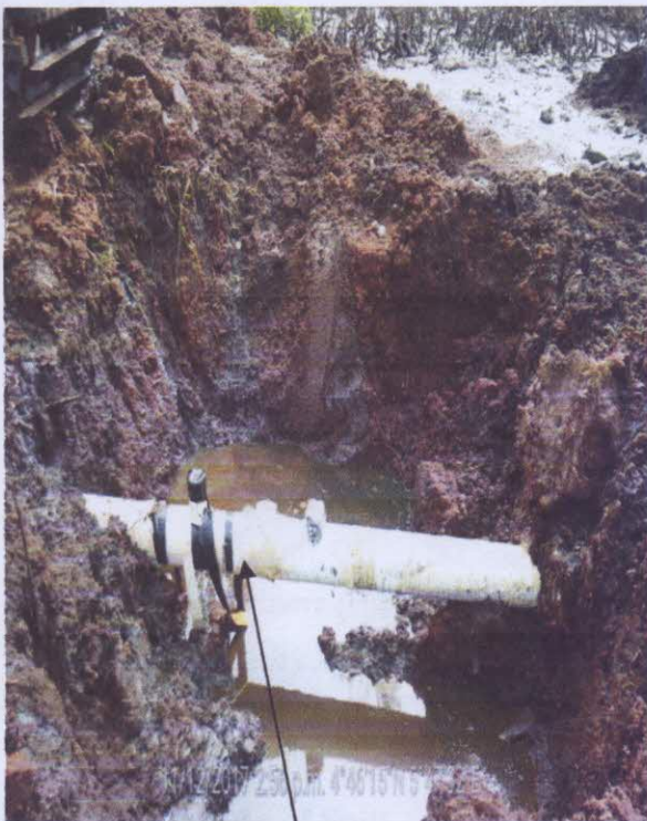
LEAK POINT AFTER REPAIR
